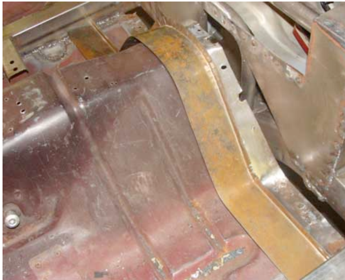
Here you can see the newly fabricated floor tunnel piece and the gap that it will fill behind it.
